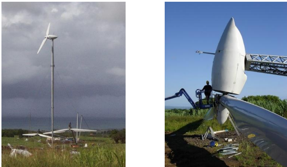
Figure 3. GEV MP 275kW in operation and tilted down for maintenance.
